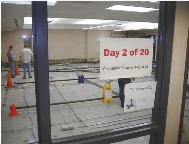
Figure 5: Demolition completed after first two days of the second phase. New network drops are visible as well as the fire-suppression system.
