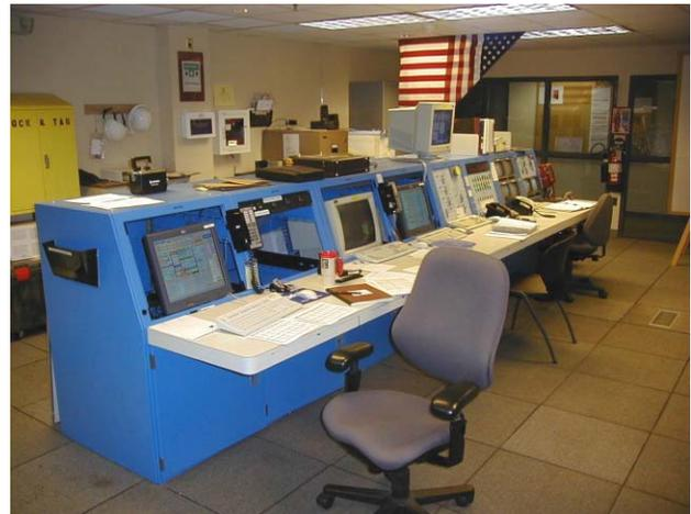
Figure 2: Safety System racks and small CRT monitors for managing accesses just visible at the far end of the console.
