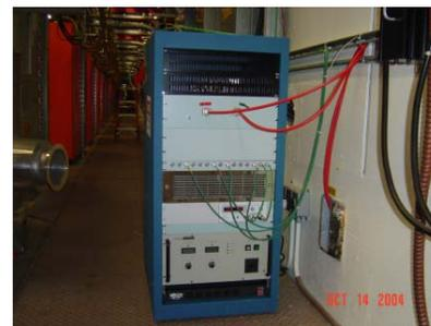
Figure 2: A barrier rf modulator in MI-60 building.
