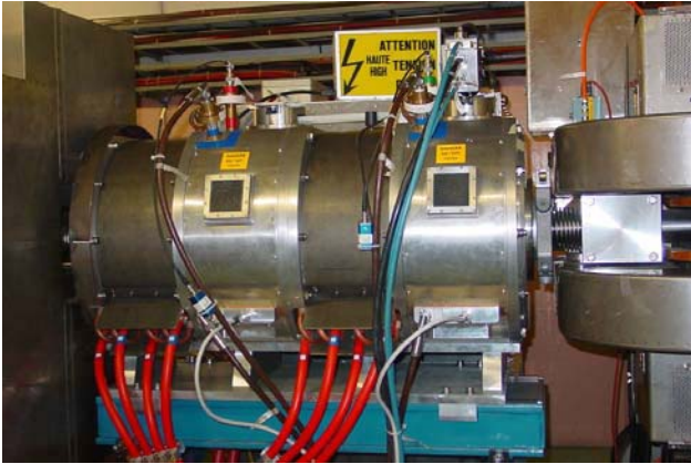
Figure 3: The cavity installed in the PS ring. The magnetic shield and the PS magnets are visible.
