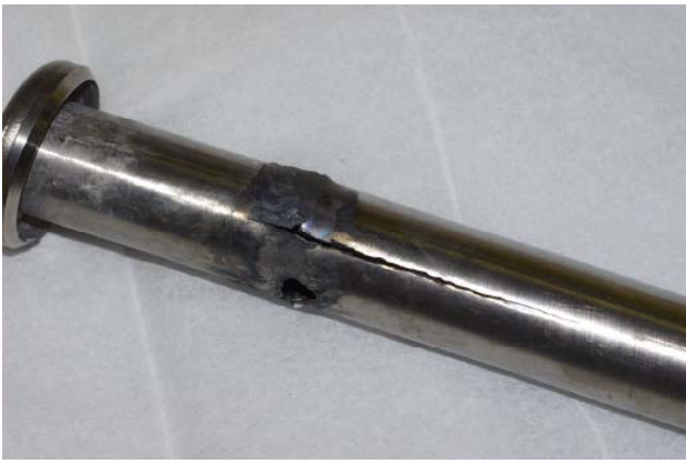
Fig. 2: Lens 21 septum conductor tube showing longitudinal crack and melted through area.
