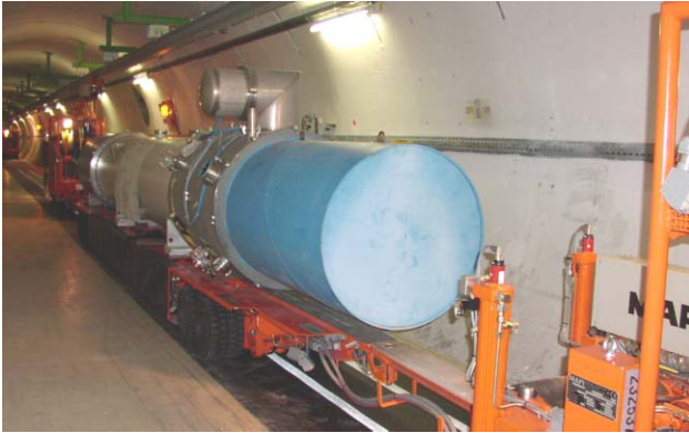
Figure 3: SSS on tunnel vehicle.
