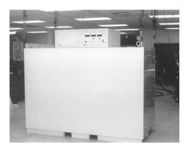
Figure 5. 140-kV, 20 A buck regulator installed at CPI.
