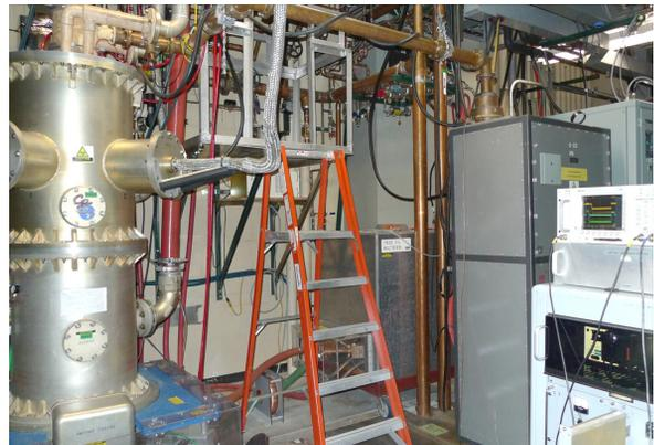
Figure 1: Old triode and tetrode RF amplifiers.
