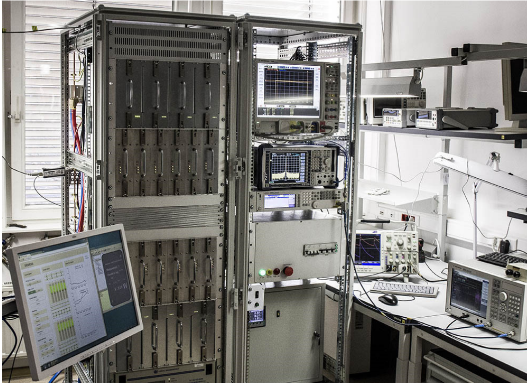
Front view of the amplifier cabinet and aux. cabinet with measurement equipment
