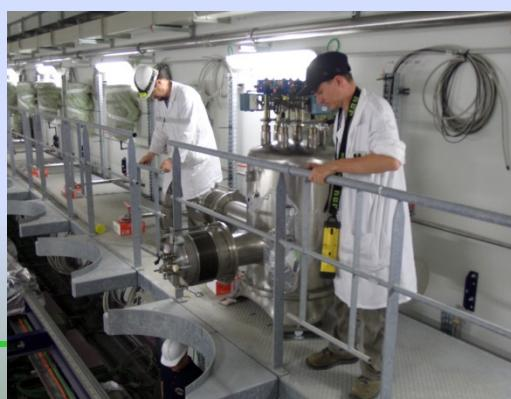
12 /12 CMA aligned and connected to their valve boxes
