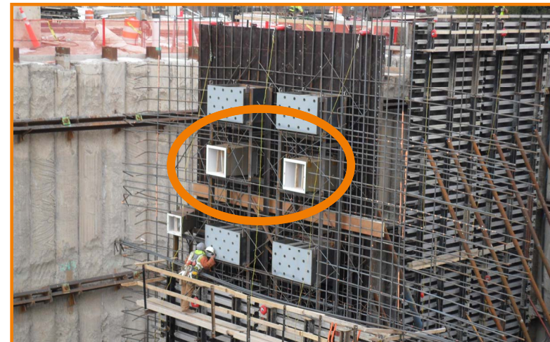
Construction verification measurements, target cell north wall alignment portal imbeds, 28 January 2015
