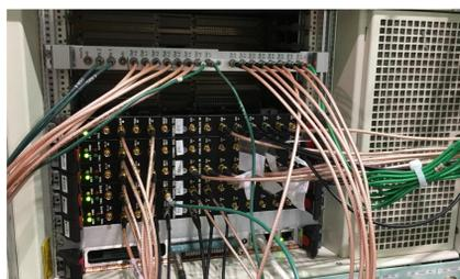
VME based electronics and timing signal fan-out
