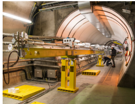
Figure 1: Picture of the vapor source 10 m-long heat exchanger under installation in the AWAKE facility. The picture is looking towards the SPS.
