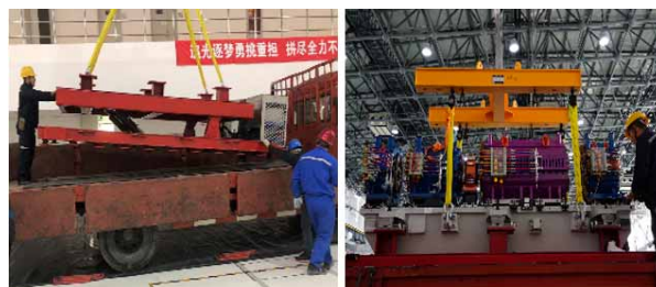
Self-levelling platform FD Unit lifted onto the truck
