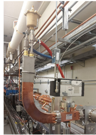
Figure 11: Vents installed on top of the RF load.
