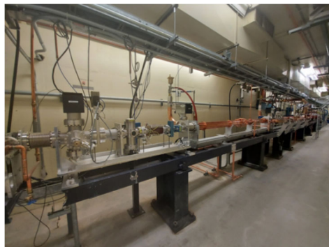
Figure 2: Overview of the new installation.
