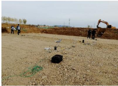
Figure 3: Graded sand and stone layer of slab #1.
