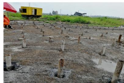
Figure 2: The prototype #4 slab: after grouting.
