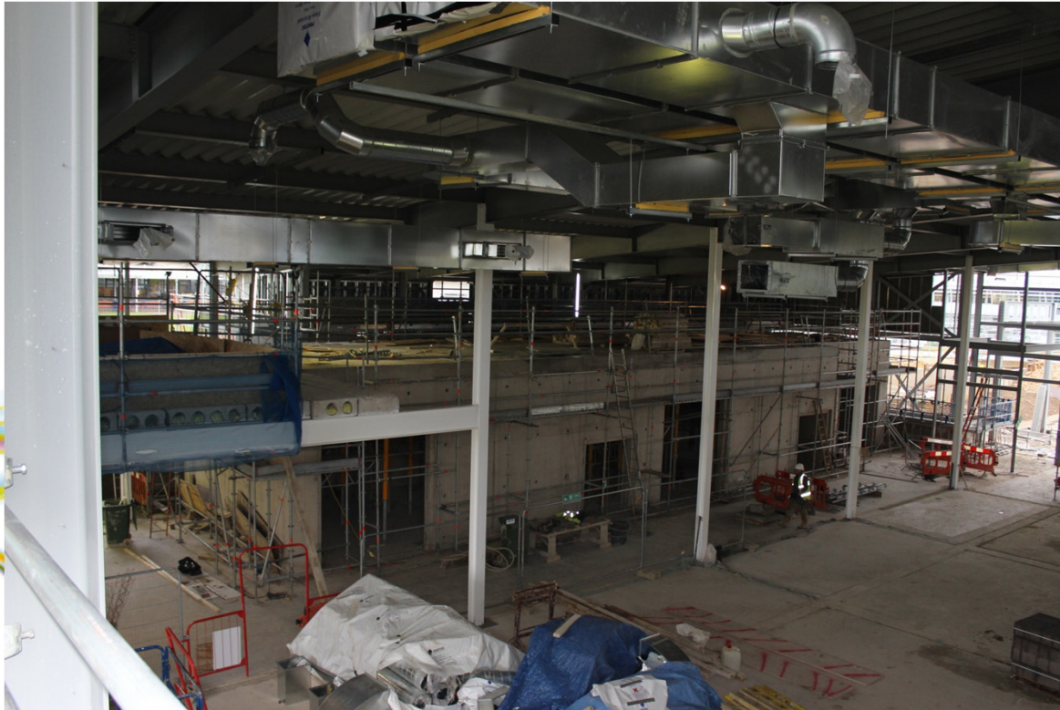
Concrete hutches under construction - Jan 2015
