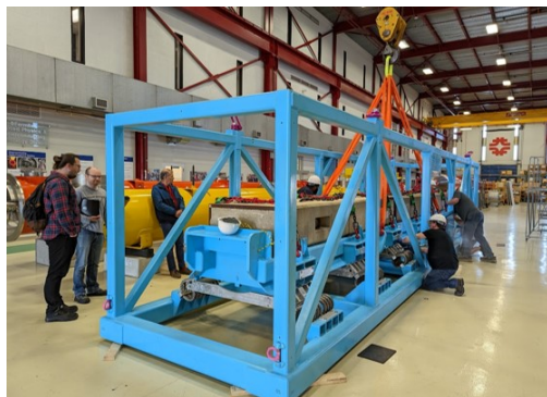
Figure 3: Transport Frame during Dummy Load installation.
