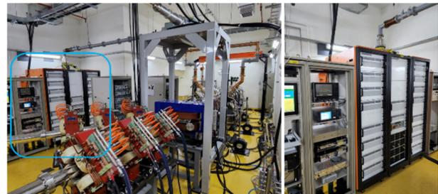
Figure 3: High power RF source installation.
