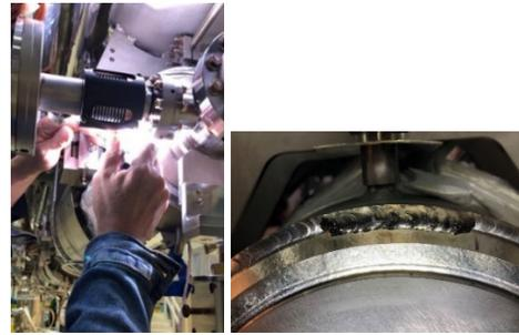
Figure 3: Helium vessel leak repair in situ on a dressed cavity during cold mass assembly.
