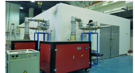
Tetrode-based RF system at site
