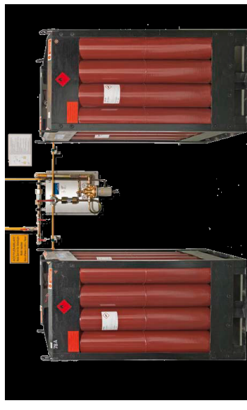
Gas supply station for cylinder bundles
