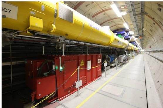
Figure 3: RF station in the E-XFEL tunnel.
