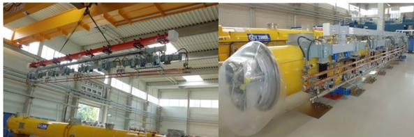
Figure 10: Waveguide installation to module.
