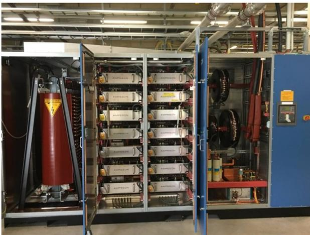
Figure 7: HV modulator.
