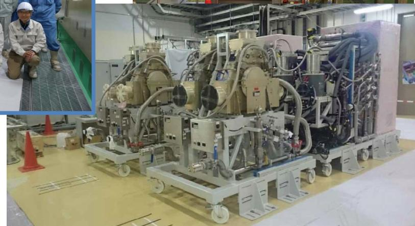
RF power system under completion
