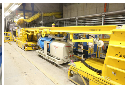
Preparation for MBK transportation inside the XFEL tunnel
