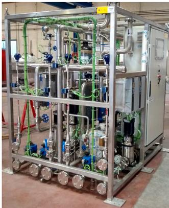
Figure 6: Picture of the cooling skid supplying chilled water to the re-buncher cavities and the scrapers.
