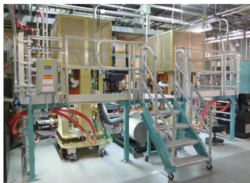
Figure 1: Dual final power amplifiers.
