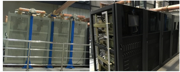
Figure 2: Two sets of 80kW solid-state amplifier.
