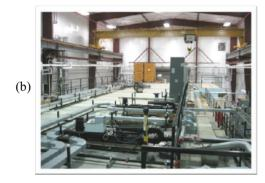
Figure 4: The expanded AWA bunker: (a) plentiful interior space is now available for the installation of the new linac tanks and new beamline switchyard; (b) new RF power circulators and waveguides have been installed on the roof of the expanded bunker, ready to connect the new klystrons to the new linac tanks.
