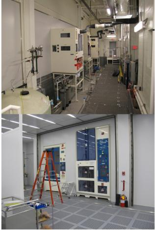
Figure 2: BCP and HPR tools bulk-headed into new cleanroom.
