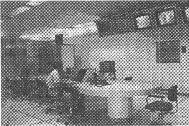
Fig. 2: View of the linac control room
