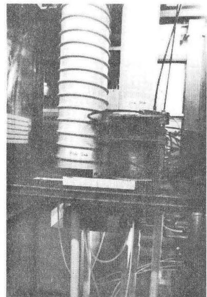
Fig. 5 Upper part of the amplifier box showing a power tube fitted with plate and grid tuning stubs.
