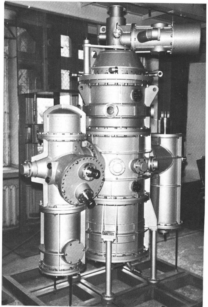
Fig. 8 First model of a power amplifier (in the mounting stage) using a grounded-grid triode.
