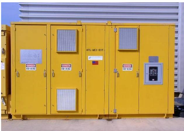
RECTIFIER TRANSFORMER AND FILTERS
