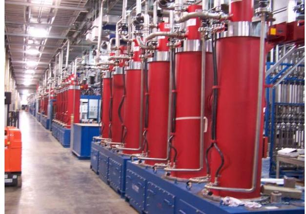
Figure 7: Klystron installation in the area of the superconducting linac. The one cavity per klystron layout requires a very dense population of rf equipment.
