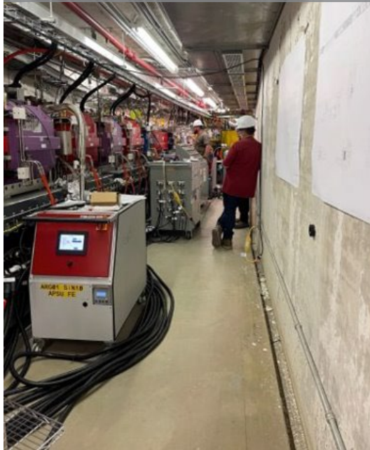
Insertion device vacuum chamber and module bakeout
