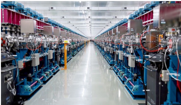
The SACLA undulator Hall [6] at RIKEN SPring-8 Center. with two 100 m rows of in-vacuum undulators
