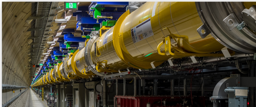
European XFEL superconducting 17.5 GeV electron accelerators (TESLA technology)
