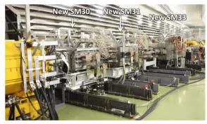
Figure 1: The high-field septa installed in MR in May 2022.
