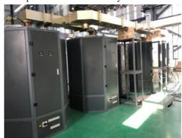
Figure 1: 650 MHz/150 kW SSA.
