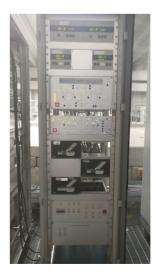
Figure 1: The TELEMA rack mounted in ALPI with MUX, PLC, ADD PLC, vacuometers and pump controllers.
