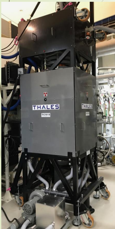
Klystron in TPS
