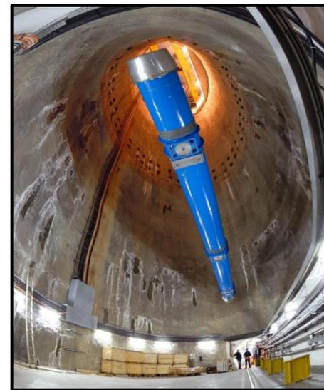
Dipole extraction from the tunnel
