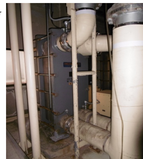
Schematic view of the cooling-water system(left) and the plate heat exchanger (right) for the PF ring.
