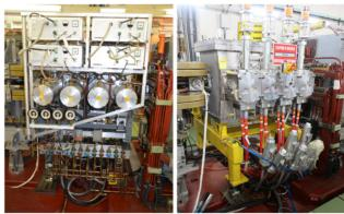
Figure 2: The old KFA45 magnet in the tunnel with s/c thyratron, TMR and oil cooling (left) and the new redesigned KFA45 in s/c configuration with the new SF6 gas free transmission cables (red) and a FC-77 filled connection box (right).
