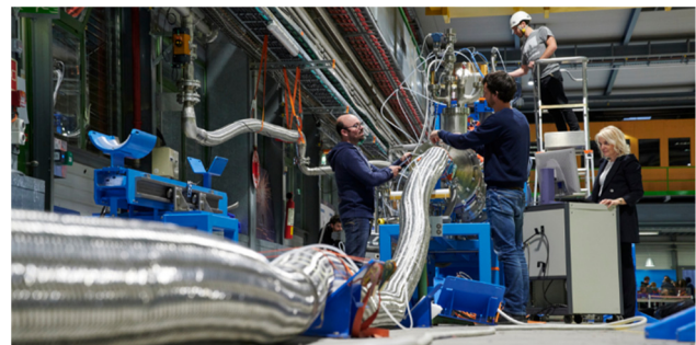
Figure 6: 60 m prototype superconducting link of 20 kA in a flexible cryostat under test in March 2019 at CERN.
