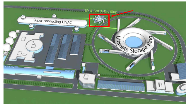
Figure 1: Blueprint of the envisioned synchrotron radiation facility. The storage ring for the EUV and soft X-rays (in red box) is presented in this study.
