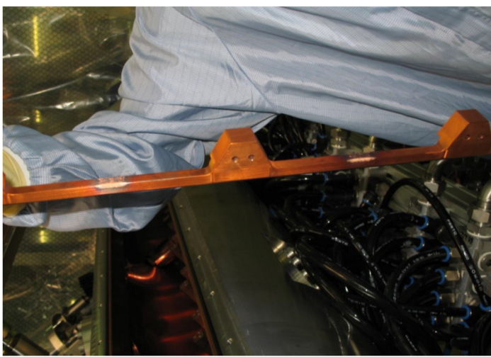
Discharge between back of the rods and stems
