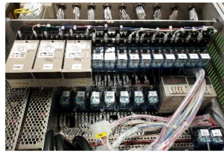
Figure 12: Redundant emergency beam trip circuits.
