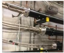
Figure 8: Output side of Blumlein generators.
