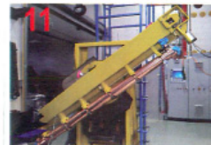
Structure reversed to horizontal position on a temporary girder
