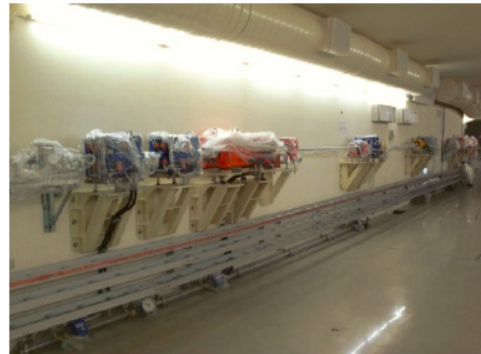
Installation of the vacuum system for the 1/12 section of booster.
