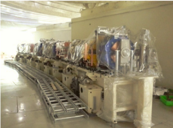
Assembling of a 14 m vacuum cell with magnets in the tunnel
