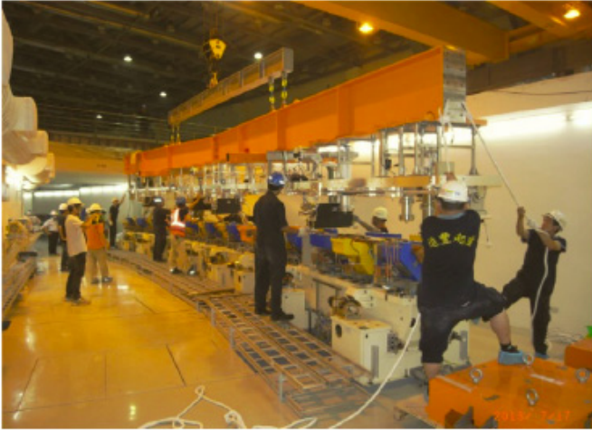
Installation of a 14 m vacuum cell on the girders.
