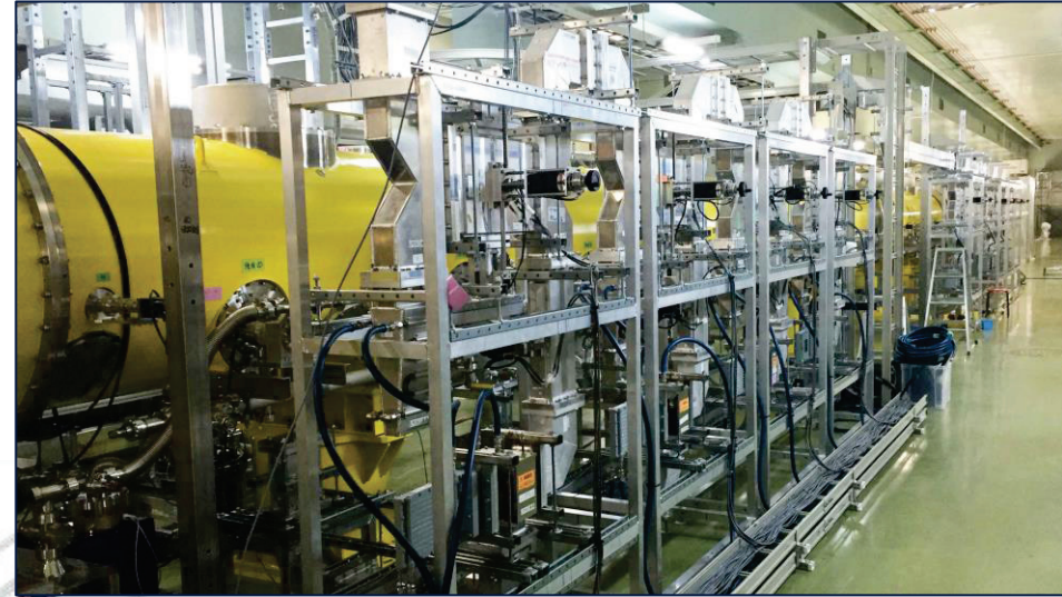
New RF power distribution (ILC-TDR design)
